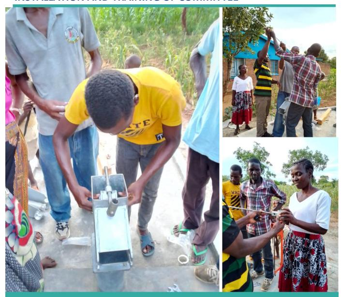
On the 11<sup>th</sup> of February, 2024 the Contractor and its technicians Installed the remaining parts of the borehole and at the same time take time to conduct a basic training for 10 committee members on borehole maintenance and repairs. The committee which is made up of 6 women and 4 men had time to do the practical training as presented in the pictures above. The training has been ongoing since day one of the project.
