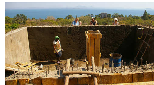
The new water tank for St Michael’s Secondary School
